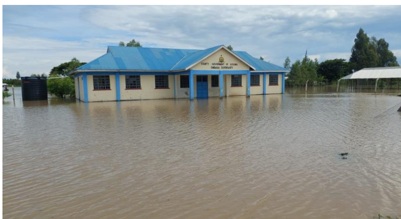
Fig. 2: A Health Facility in Nyando Sub County in Kenya Submerged in the Floods
